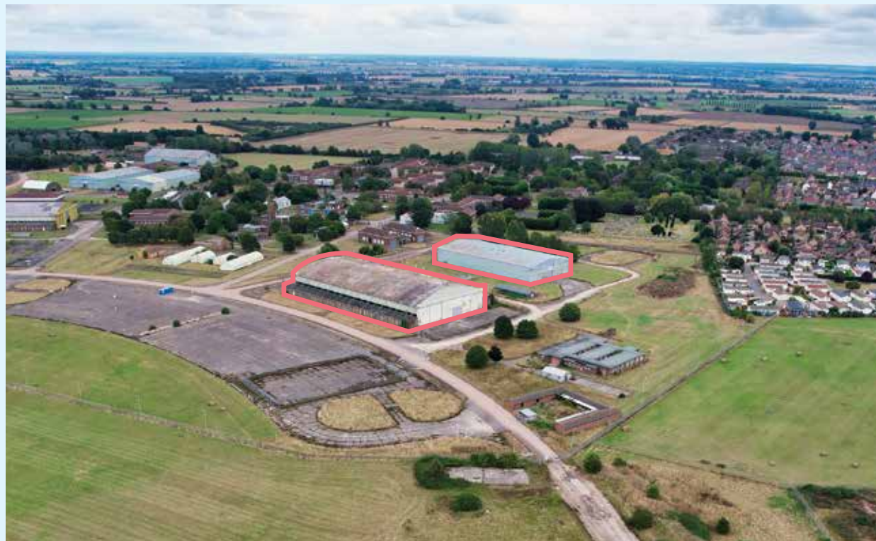
Southern hangars scheduled for demolition late January/early February
