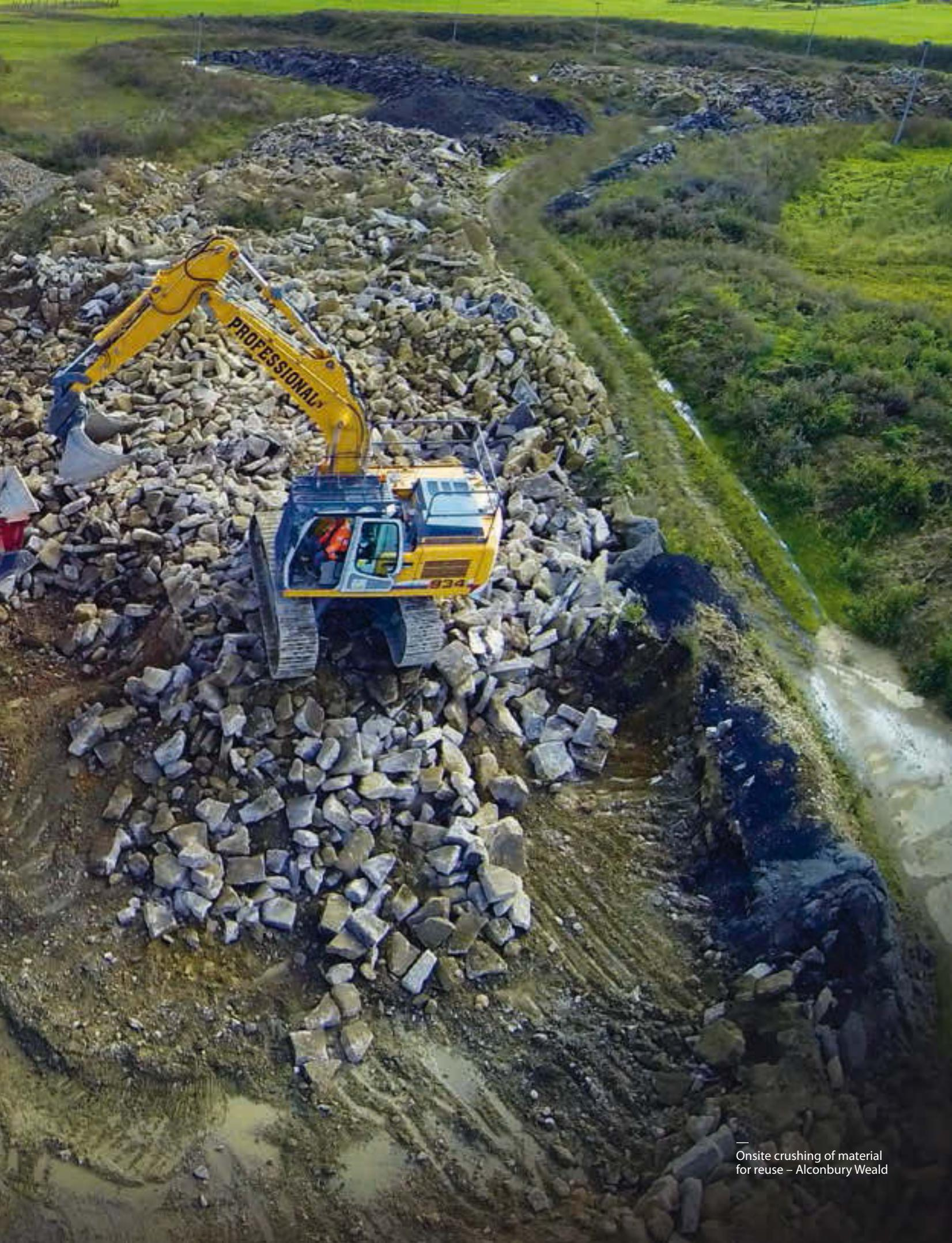
Onsite crushing of material for reuse – Alconbury Weald
